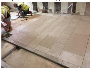
clearly defined layout. You can also see how the tiles bridge over the cable ducts.
