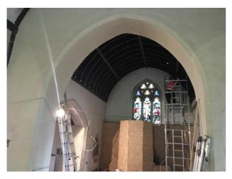
Work has now started on laying the stone floor tiles. There was a bit of a delay while the electricians took over virtually the whole site, working at both high and low level. By the end of the week they had pretty much completed their 'first fix'. The picture shows them putting cables in the Chancel ceiling which was the last part to be completed.
